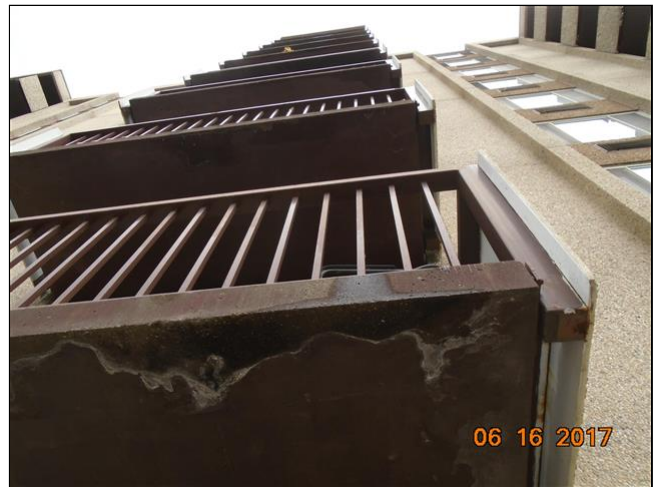
4.1 Item 4(Picture) Decks are structural cement panels- There was some water staining-but no structural issues could be found.
