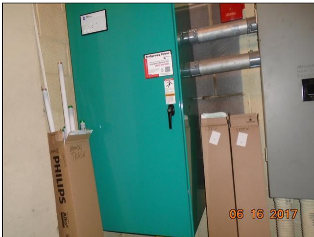
8.0 Item 8(Picture) Cummins Transfer Switch
