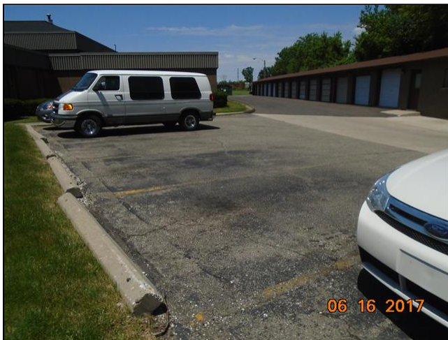
3.0 Item 9(Picture) Employee parking-only small areas of asphalt need repair
