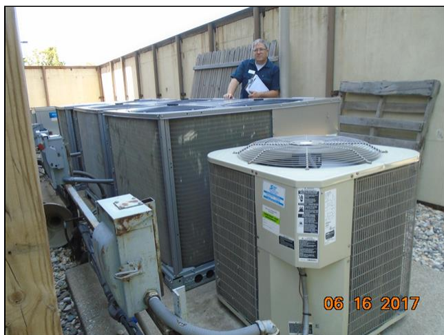
6.0 Item 12(Picture) Outside air condenser fins were clogged, and had hail damage.
