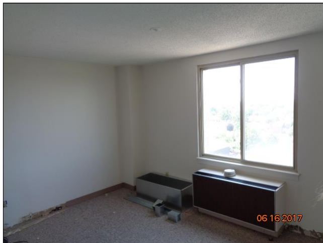
6.0 Item 8(Picture) The framework for the new Amana replacement needs to be retrofitted to adapt to the smaller new units.
