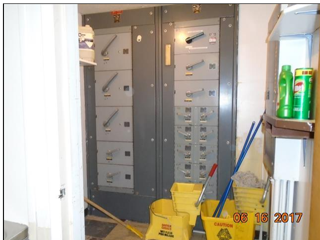
7.0 Item 1(Picture) Aged switchboards require a maintenance plan
