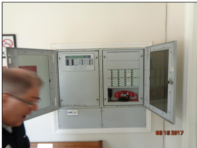
8.0 Item 1(Picture) Basic alarm control center requires stall location of triggered smoke alarm
