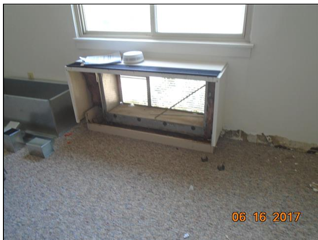
6.0 Item 9(Picture) The framework for the new Amana replacement needs to be retrofitted to adapt to the smaller new units.
