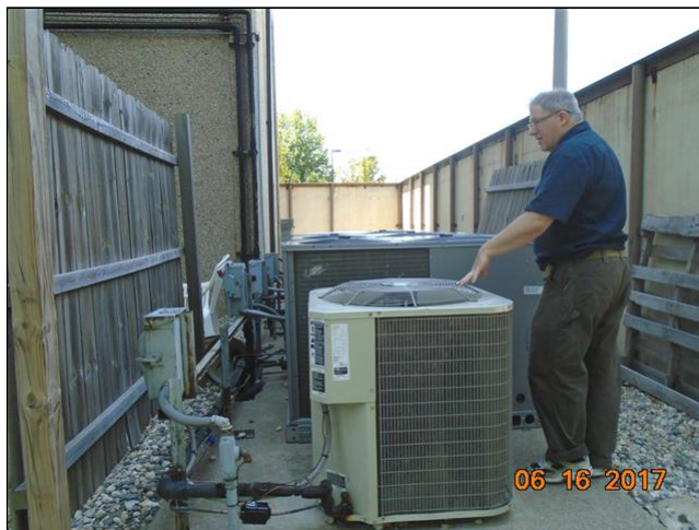
6.0 Item 11(Picture) Outside air condenser fins were clogged, and had hail damage.
