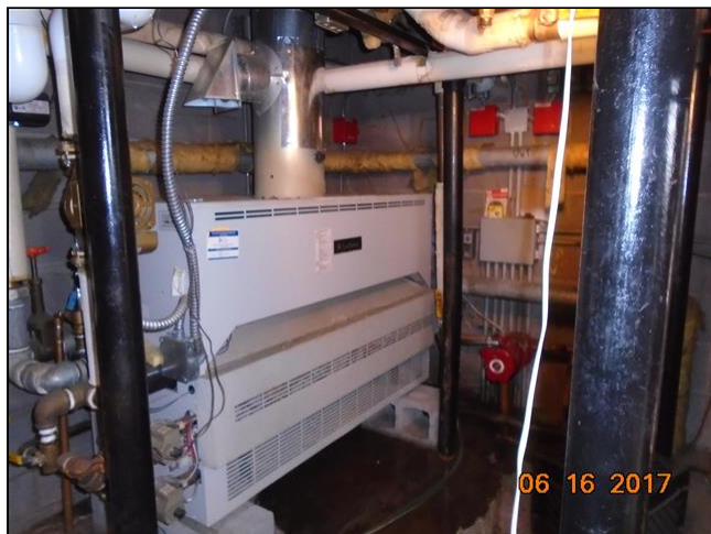
5.1 Item 1(Picture) Water on floor below Lochnivar boiler- needs service
