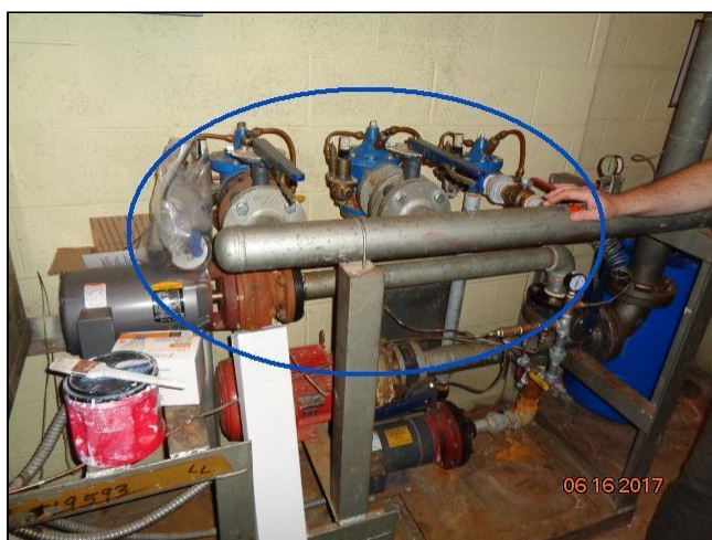
8.0 Item 3(Picture) Three new Pumps to send sprinkler to upper floors
