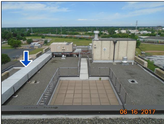
6.0 Item 3(Picture) AHU duct return and supply vents at each end of hallways 3-10-great condition
